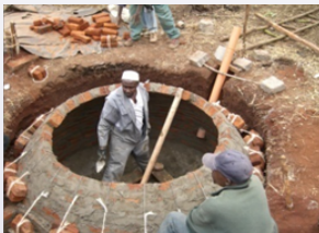
Construction of biogas units for households in Kenya
